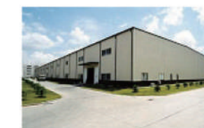
厂房土建 PLANT CIVIL CONSTRUCTION
